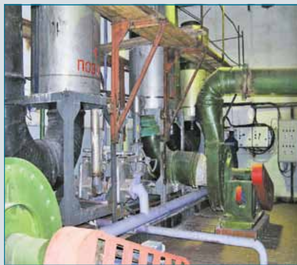
The neutralization section of JSC "Buryatzoloto" gold-mine "Holbinskiy" hydrometallurgy workshop (performance 500m 3 /day)
